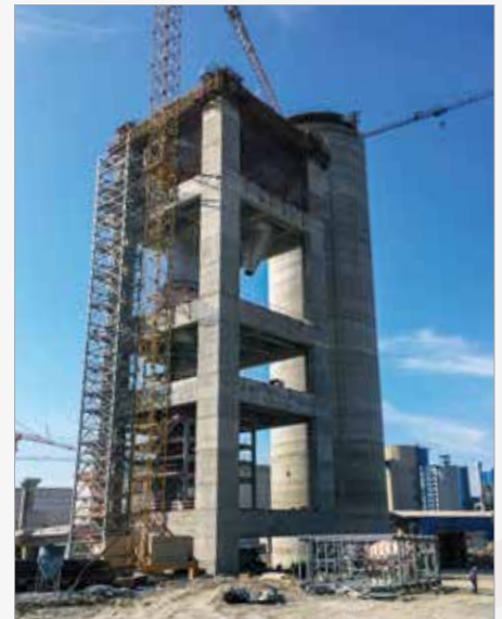
Concrete Pumping at 175 m Height
